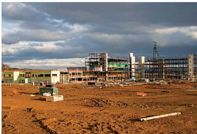
Work on the steel structure comes into place in March 2008.
